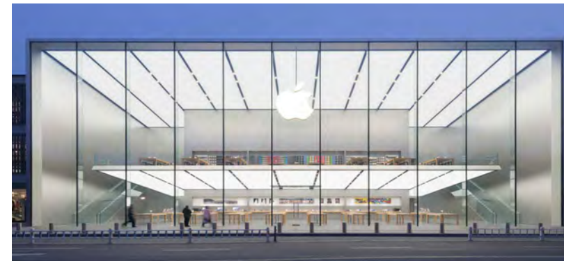
The state-of-the-art Apple Flagship Store's entire rooftop is equipped with a SKYCO Skylights photovoltaic (BIPV) system to offset power consumption.
