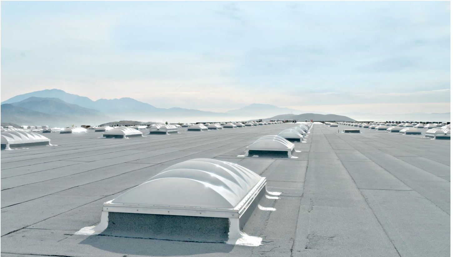
The FM Approved 4x8 Industrial Skylight by Skyco Skylights is an extreme wind uplift rated (195 psf), super strong polycarbonate dome unit skylight.
